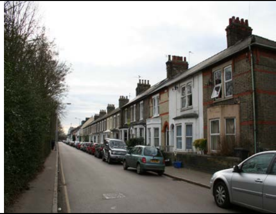
Brick detail painted over.
